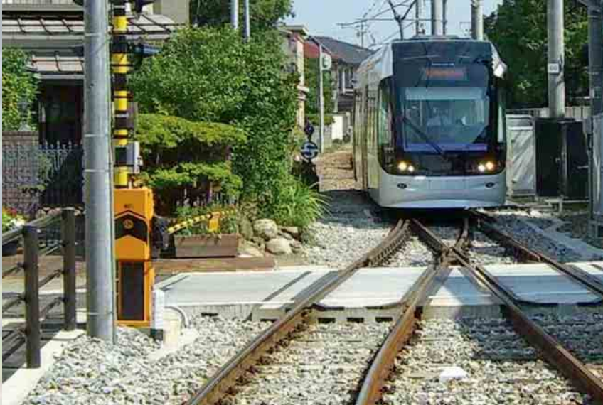
Single-line track safety devices
